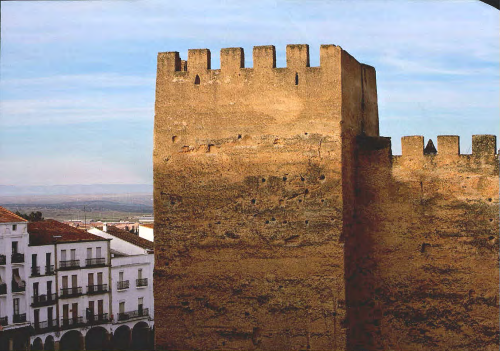
Yerba Tower wall, Cáceres
